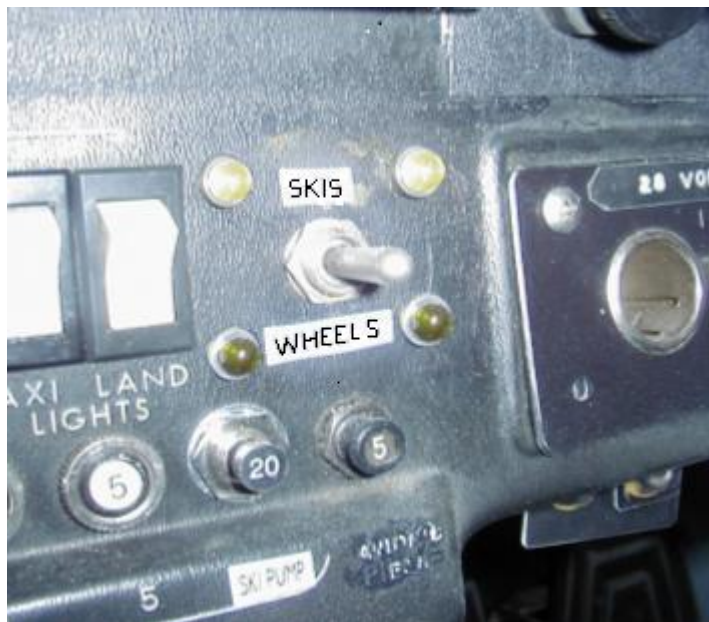
Ski Pump Switch Installation-Photo 8
