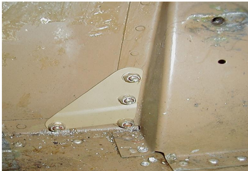
Rear Rigging Bracket Doubler Installation LH3600-17-1 (LH3600-18-1 Opposite) Photo 3
