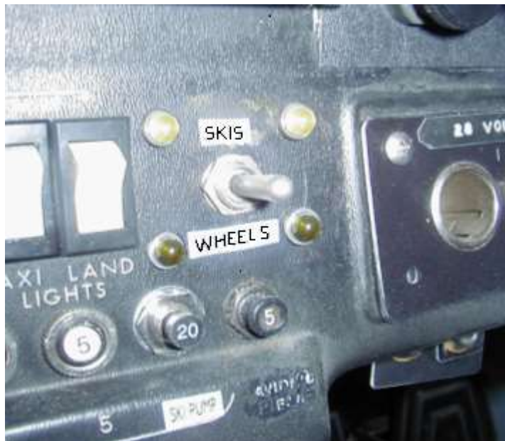
Ski Pump Switch Installation-Photo 7
